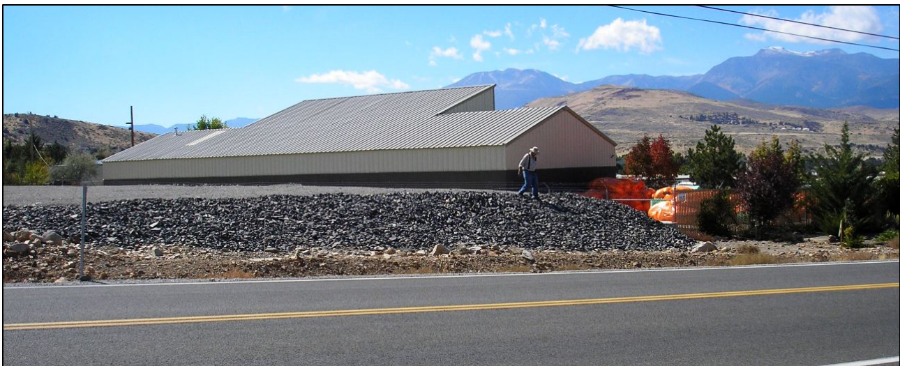
View of Existing Structure (NE corner of property) from Across Geiger Grade (photo courtesy of Sonoran Roofing)
