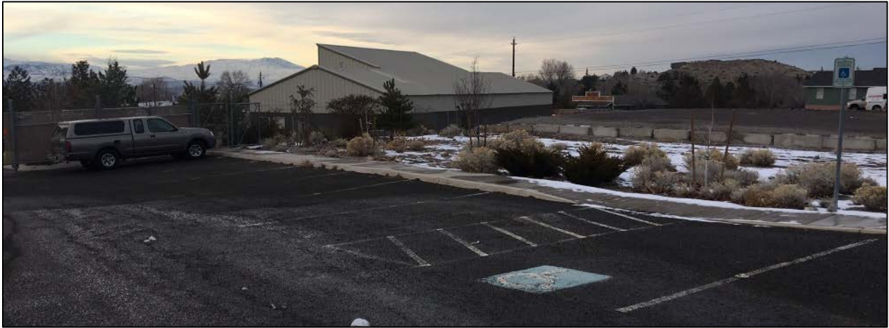
View of Existing Structure from Kivett Lane Entrance
